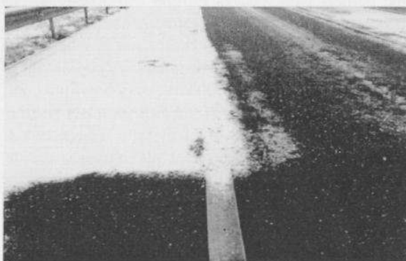
Hard shoulder of porous asphalt next to dense asphalt concrete road surface. Shoulder is fully covered with snow because without traffic action, salt remains in voids rather than transferring to surface.
